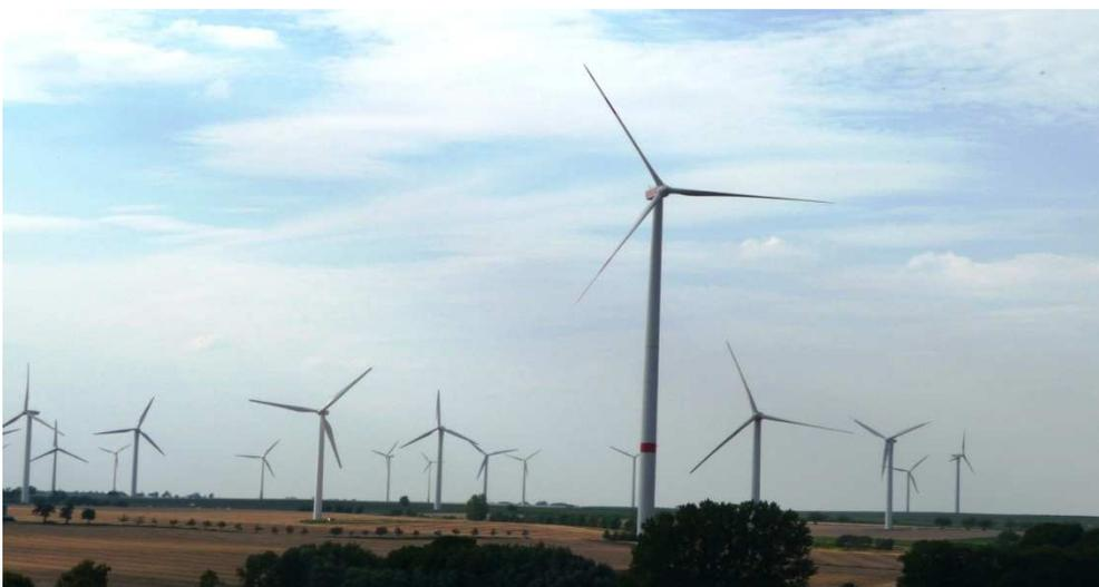
Abb. 3.2.2-2: WEA Typ Vestas V 90-2MW (P = 2 MW; NH = 125 m; RD = 90 m)
