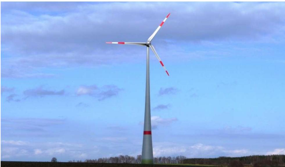
Abb. 3.2.2-1: WEA Typ Enercon E 82-2MW (P = 2 MW; NH = 138 m; RD = 82 m)
