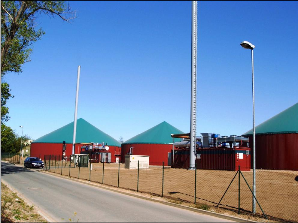
Abb. 3.3.4-3: BGA Großenhain (MEI) – 2 BHKW -  $P_{\text{Net}} = 2 \times 716 \text{ kW}$ ,  $P_{\text{Nth}} = 2 \times 700 \text{ kW}$
