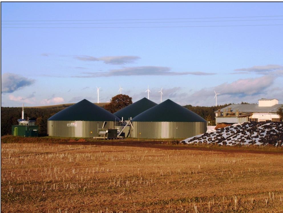
Abb. 3.3.4-4: BGA Reinhardtsgrimma (PIR) – BHKW  $P_{\text{Net}} = 500 \text{ kW}$ ,  $P_{\text{Nth}} = 500 \text{ kW}$
